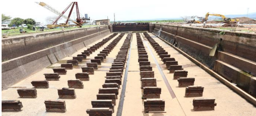
Fig. 9. Preparation of dry Dock prior for MV Uhuru II Construction
