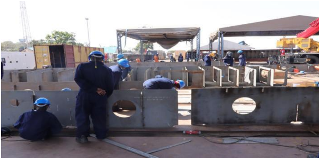
Fig. 12. Fabrication of the sections
