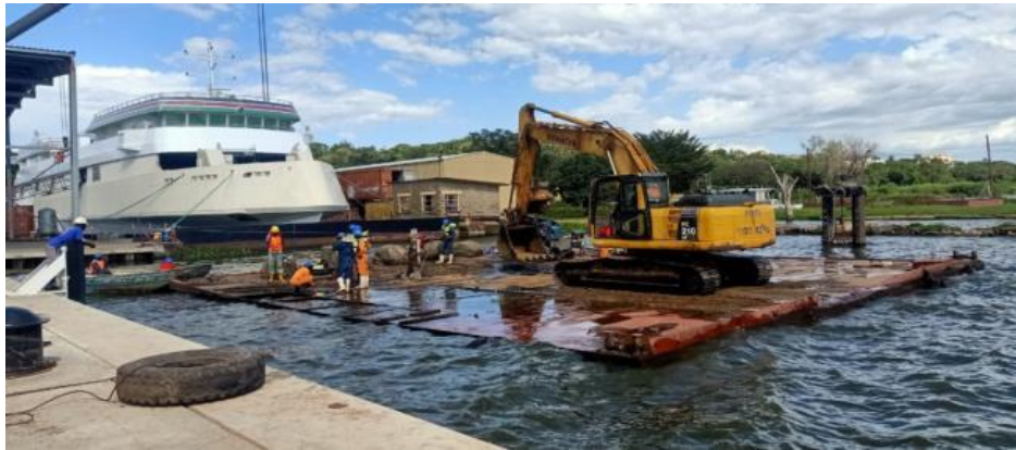
Fig. 3. Dredging work at dry dock frontage
