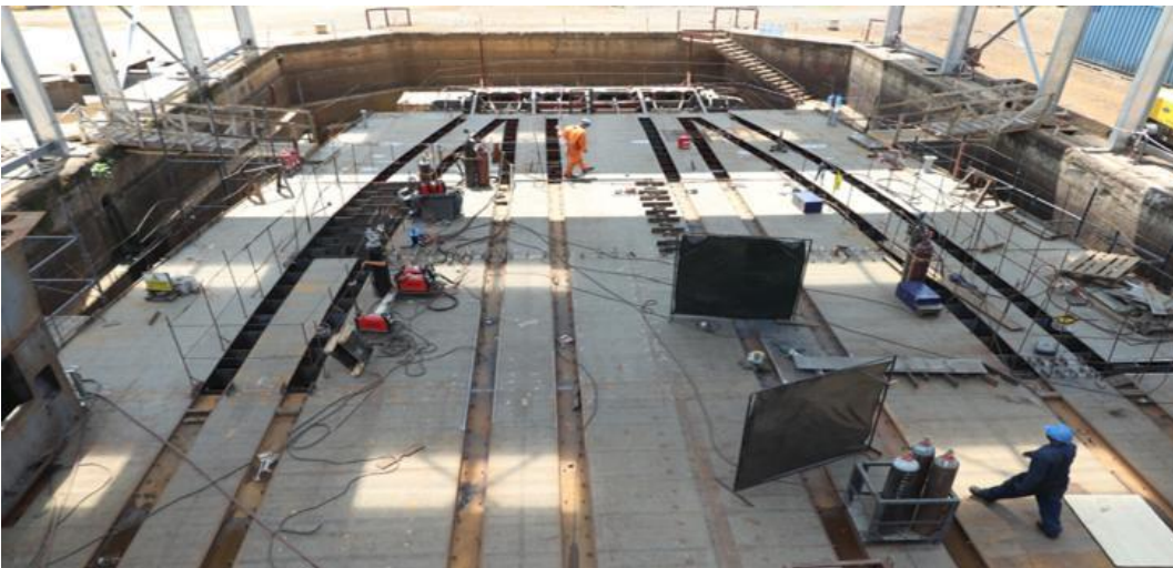
Fig. 16. Construction of bridge deck
