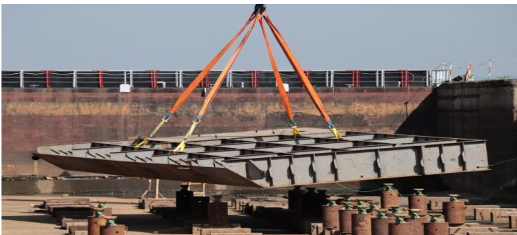
Fig. 14. Installation of first section
