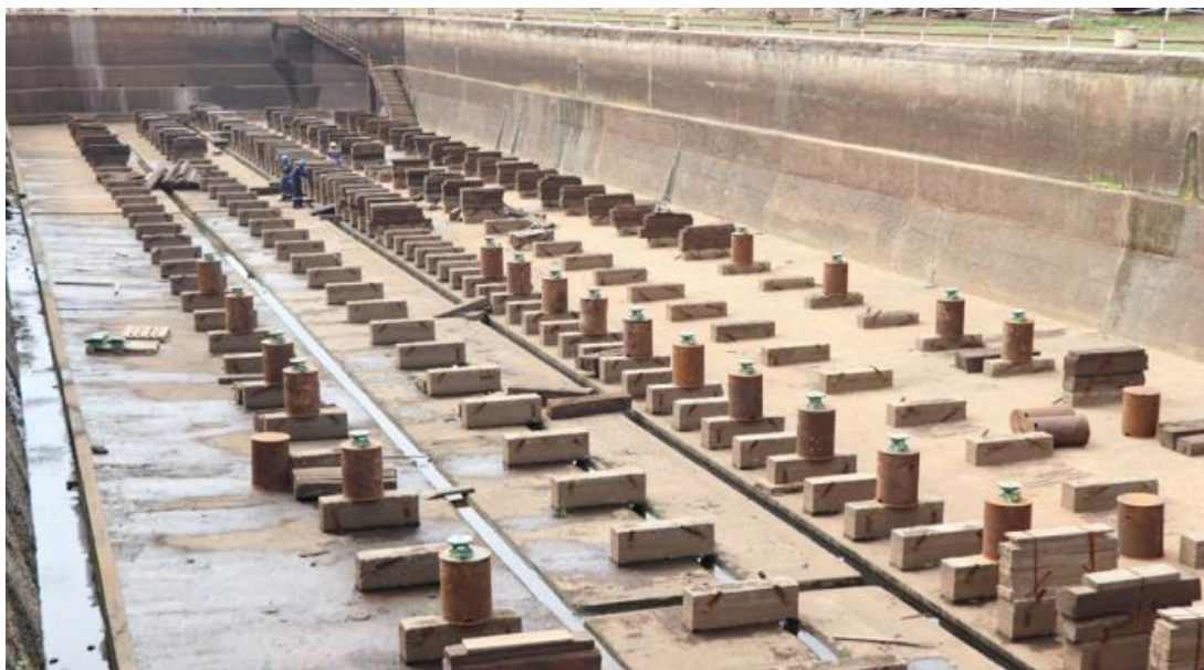
Fig. 11. Installation of Keel blocks and pipe stand
