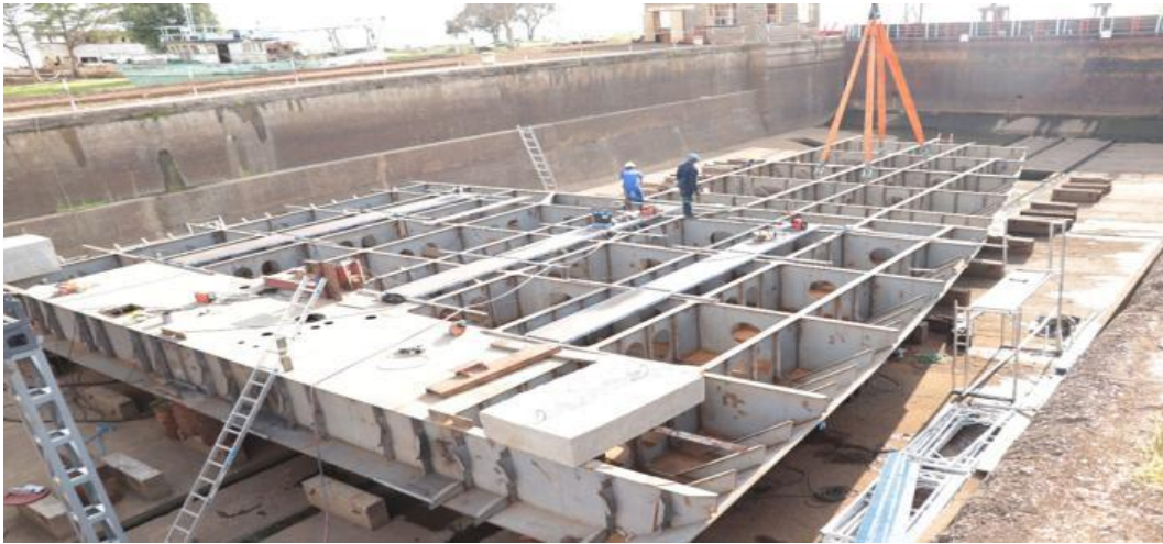
Fig. 15. Installation of upper deck section
